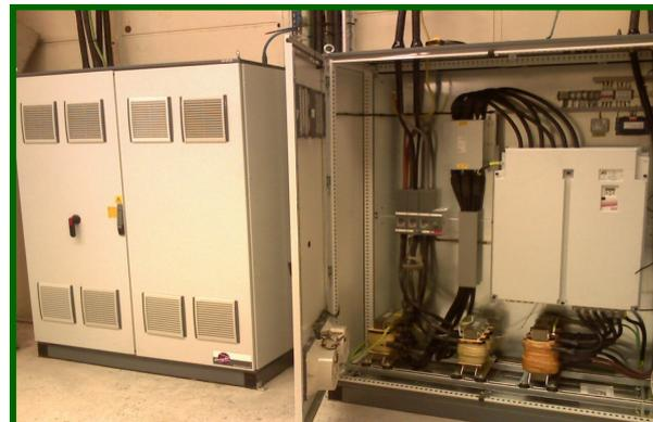
Variable Speed Drive for 300kw Piston Compressors
