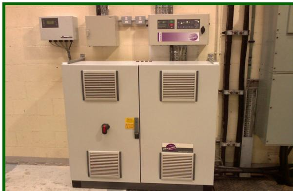
Variable Speed Drive for 75kw Screw Compressors
