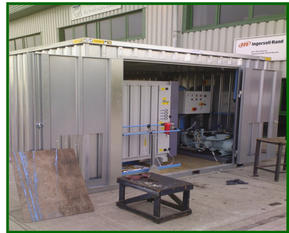
Inside the plant room
